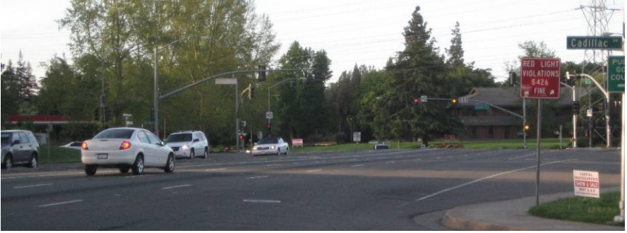
Southbound on Howe Avenue:
