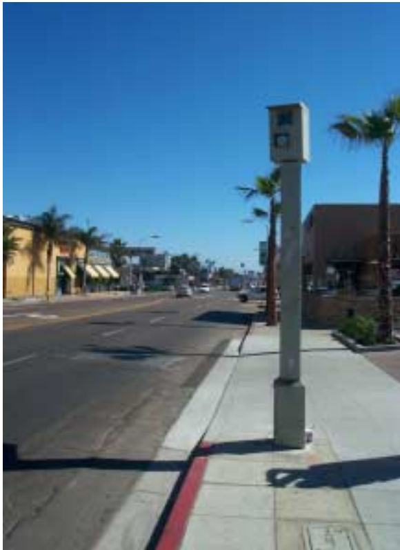
Figure 4-1 CAMERA POLE AND HOUSING
