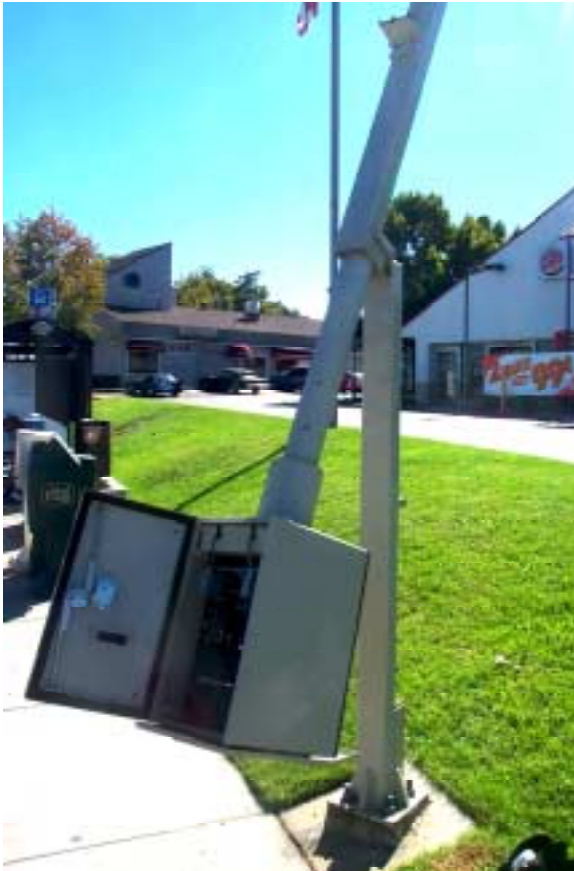
Figure 4-4 LOWERED HINGED POLE
