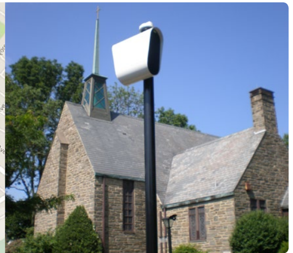
RLC installation @ Old Welsh & Old York - Abington, PA
